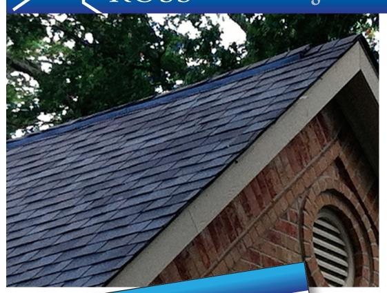
The Ross 2-IN-1 Ridge Vent is a patented product with many design innovations. The Ross 2-IN-1 comes standard as a 12" but can be converted to fit 9" cap shingles, as well as 10" cap shingles, by scoring the underside groove opposite the cut break line on top of the vent. The Ross 2-IN-1 offers 84 Square Inches of Net Free Area and is GREEN.
